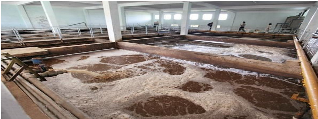
Figure 4: Latex septic tank
